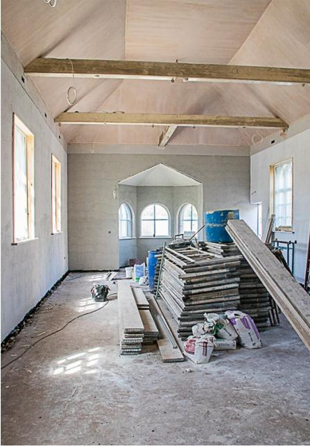
The builders, Trio are still cracking on at a pace and making a great job of it, the foyer, toilets and kitchen are all plastered and the kitchen units are being fitted as we go to press. The main hall has to be plastered with lime plaster - a three layer process. It has to cure between layers. The first coat had been applied when these photos were taken. Trio's expectation to finish is still by the end of July and we can't wait to see it.
